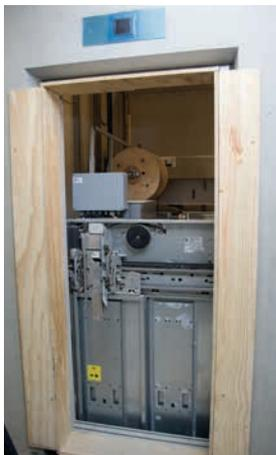
***KONE construction time elevators** are the final elevators equipped with protective materials so they can be used during construction time. They operate at the same speed and load as the final elevators. When the building is finished the final signalization and interior are installed in the elevators.*
